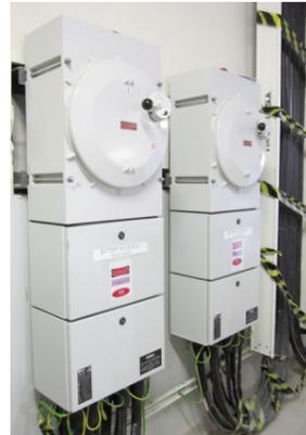
Explosionproof switchgear assembly type SAd / GHG
